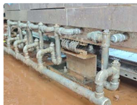
Heating Ventilation and Air Conditioning (HVAC) Drain Pipe Installation
