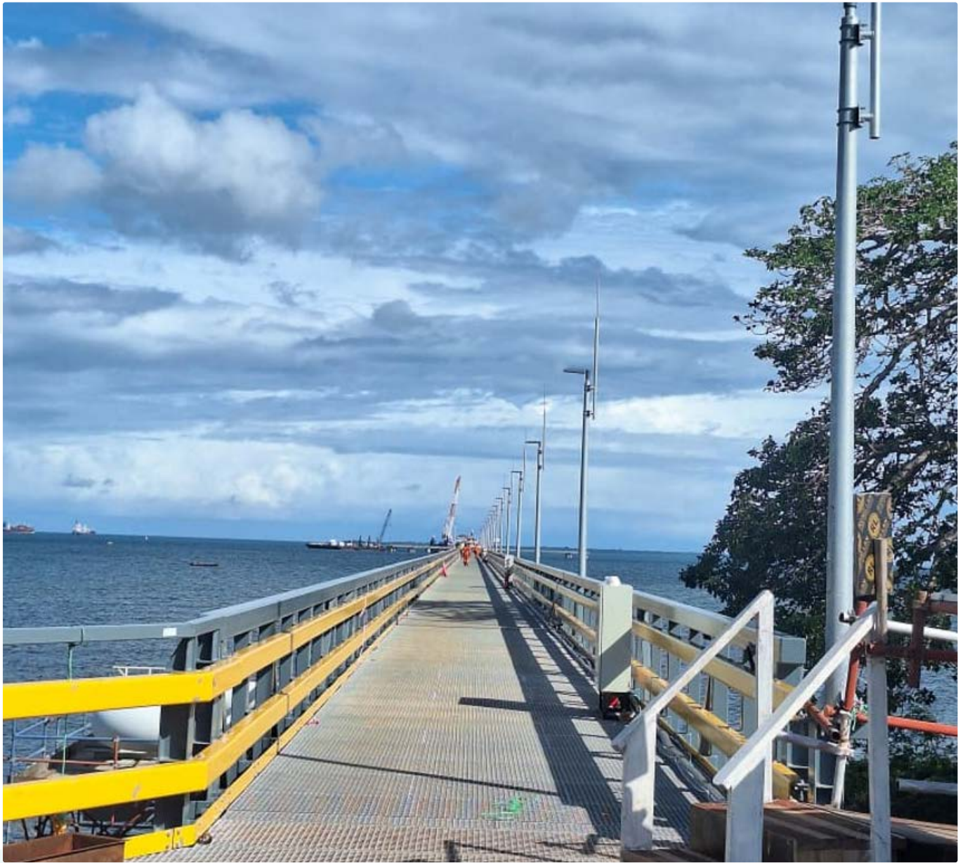
Lighting Poles Installation
