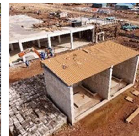
Office Building Roof Concrete Casting
