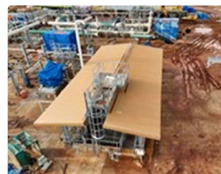
Closed Drain Drum (CDD) Structure Installation
