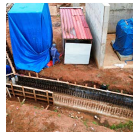
Formworks for Outside Diameter-03
