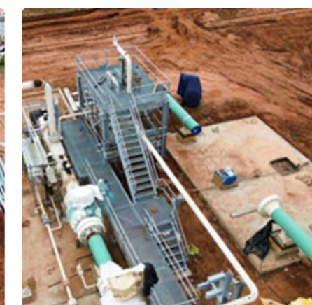
Pig Receiver Structure Installation
