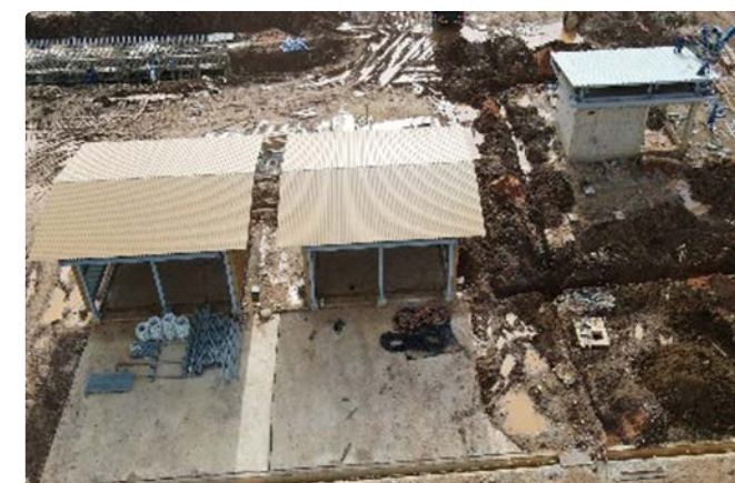
Chemical Injection Shelter Installation
