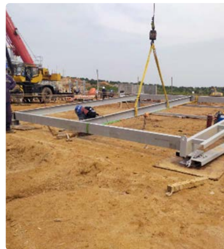
Steel Structure Erection
