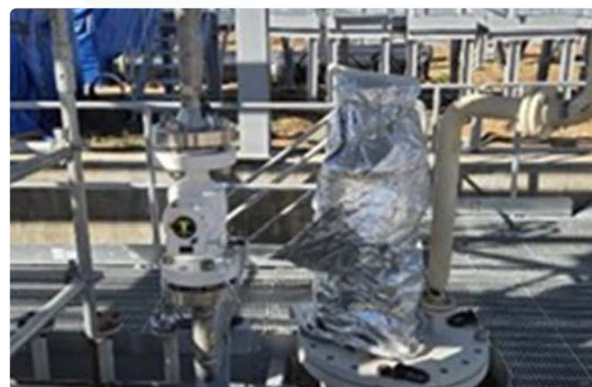
Process Pipe Welding
