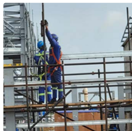
Cable Tray Installation
