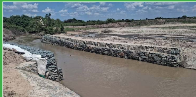
Construction of gabion walls at the crossing for long-term erosion control and stabilization
