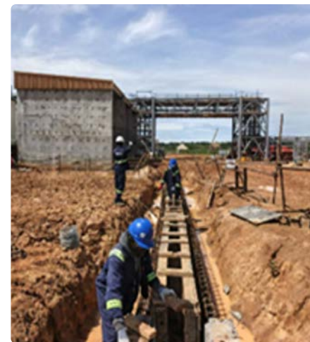
OD3 Trench Formwork
