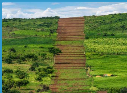
View of the ongoing buried pipeline reinstatement process along the EACOP Right of Way.
