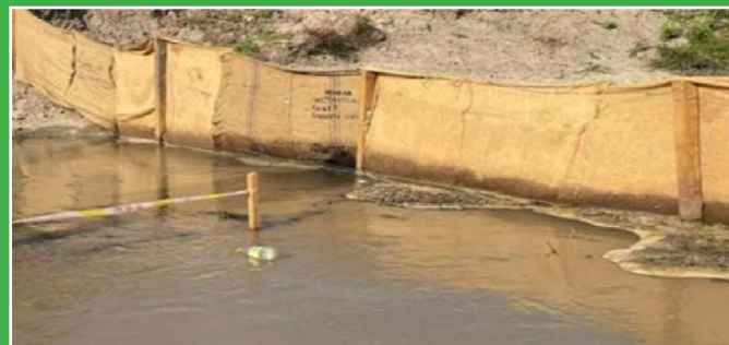
Silt trap installed downstream of the crossing
