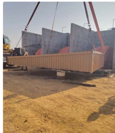
Transformer Shelter Erection
