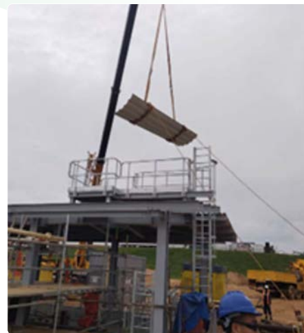
Closed Drain Drum (CDD) Roof Erection
