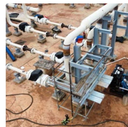
Cable Tray Support (CTS) Structure Welding
