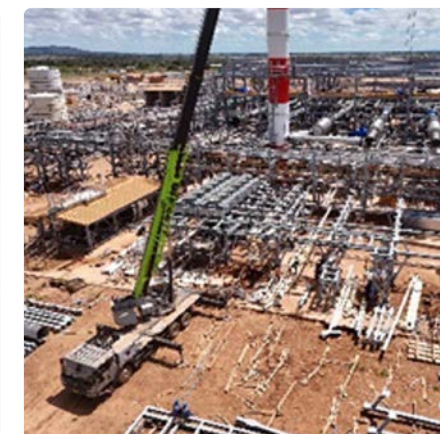
Radiator Structure Installation
