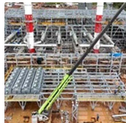
Radiator Structure & Radiator Installation
