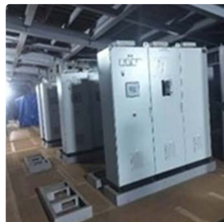
Low Voltage Switch Gear Installation
