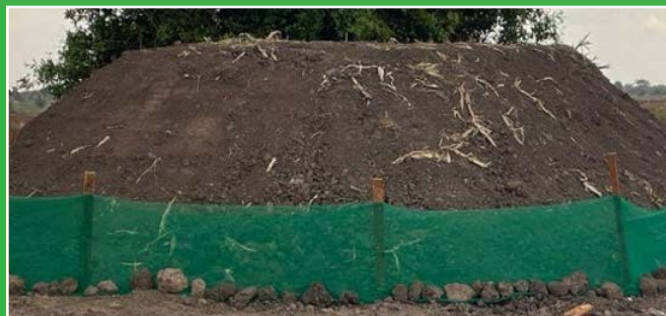
Protection of stripped topsoil from diversion channel
