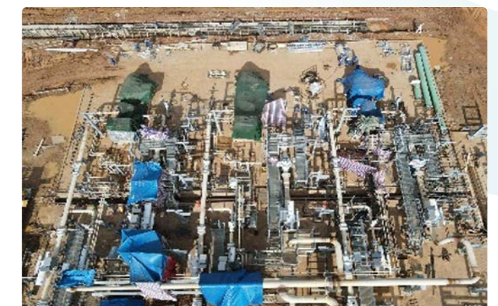
Piping pool Installation
