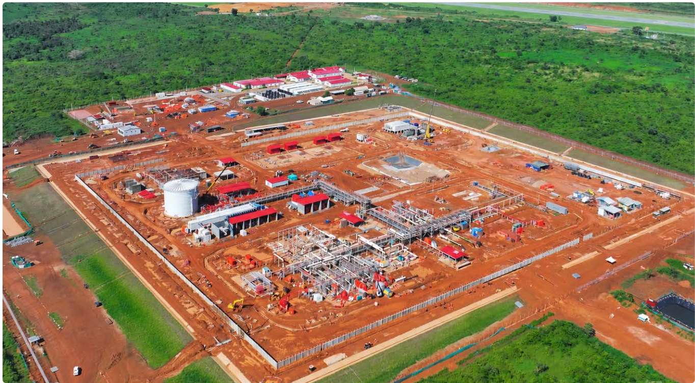
Pumping Station 1 (PS-1) Aerial View
