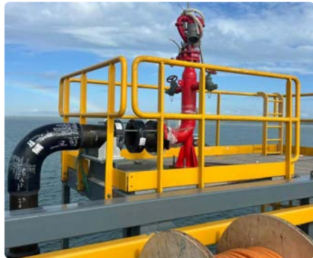
Fire Hydrant Installation
