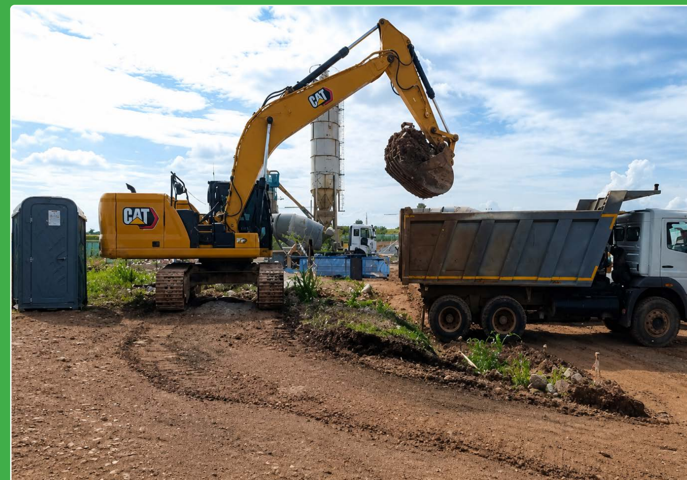
Loading and transportation of unused concrete waste
