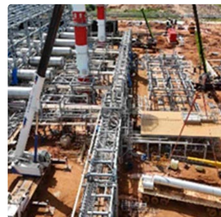
Power Generation Building (PGB) Exhaust Duct Installation
