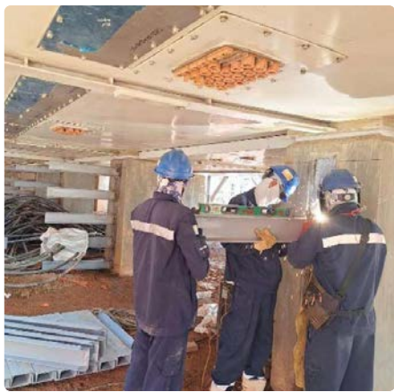
Tray Support Installation Below 33kV Electrical, Instrumentation, Telecommunication and Security Systems (EITS)
