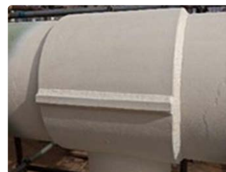
Coating of Pipeline Support
