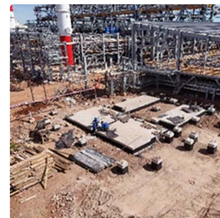
Electrical, Instrumentation, Telecommunication and Security Systems (EITS) Transformer Roof Installation
