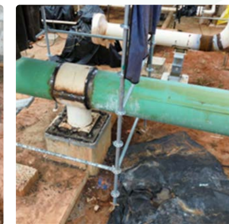
Pipeline Supports Welding
