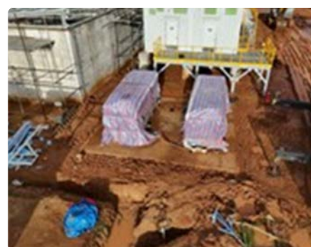
Heating Ventilation and Air Conditioning (HVAC) Unit Installation
