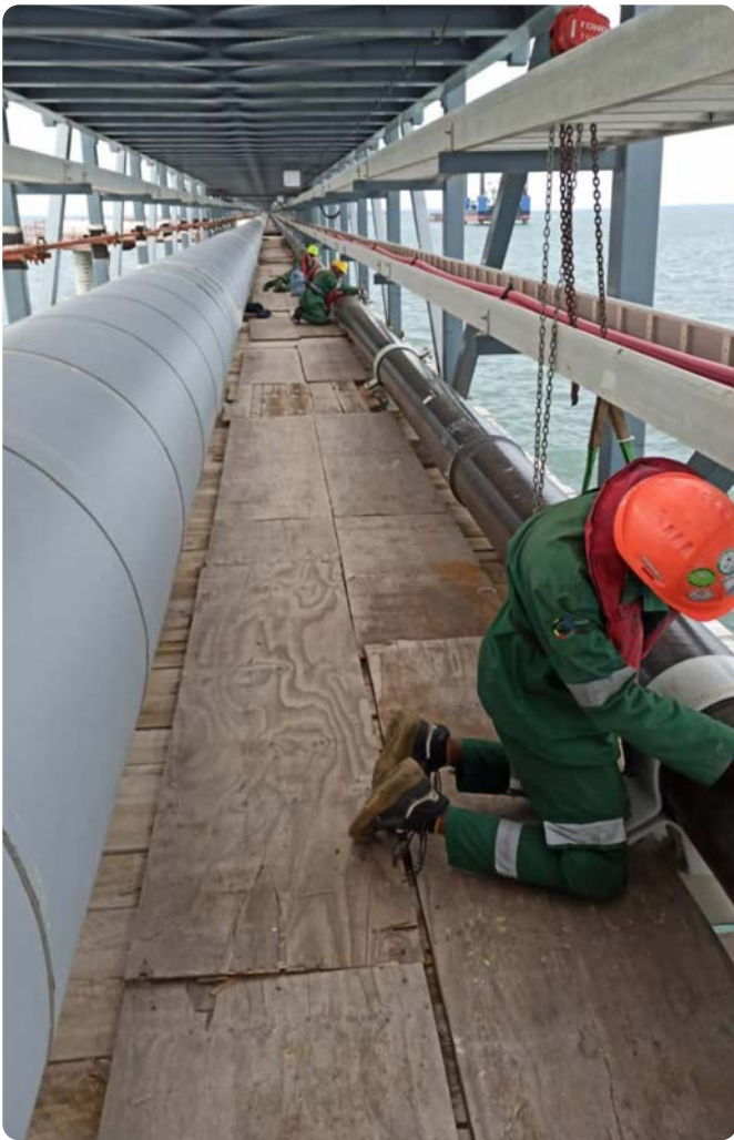
Glass Reinforced Epox (GRE) pipe bonding & clamping
