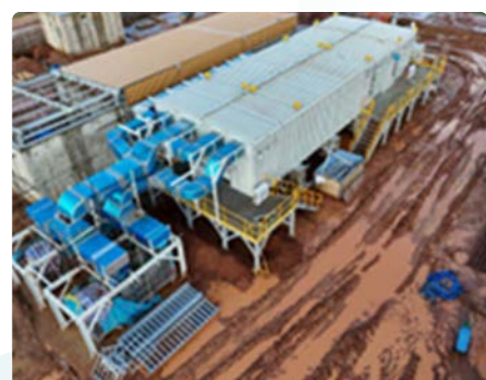
Electrical, Instrumentation, Telecommunication and Security Systems (EITS) Installation
