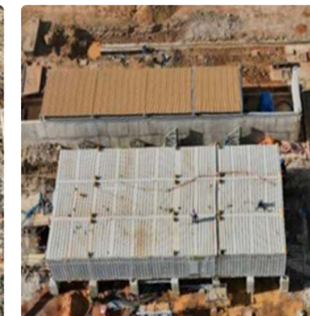
Electrical, Instrumentation, Telecommunication and Security Systems (EITS) Building Installation
