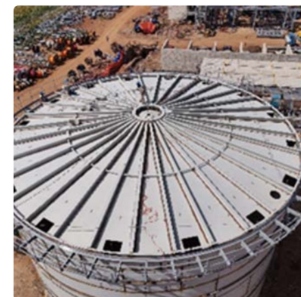
Fire Water Tank Roof Accessories Installation
