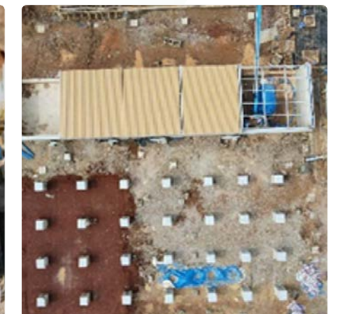
Transformer Roof installation
