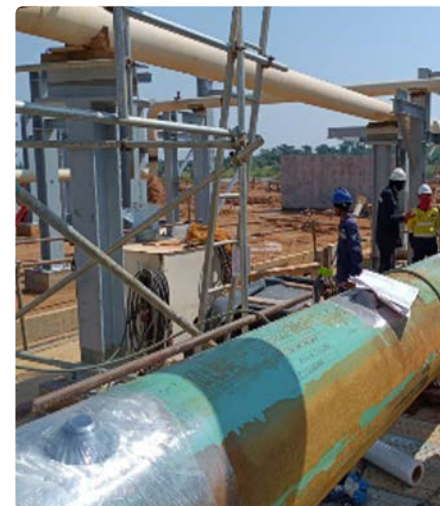
Piping Work in Progress
