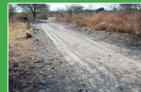
Rehabilitated the community road section after completion of works
