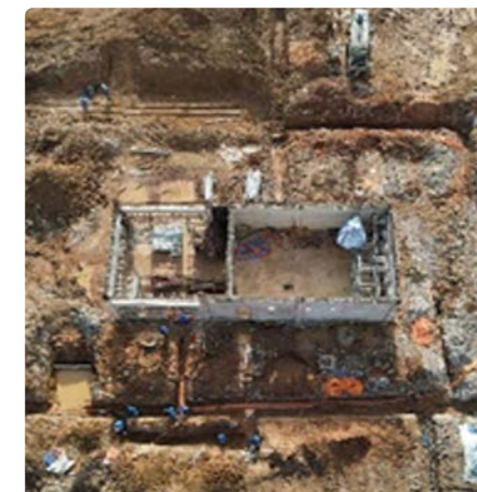
Electrical, Instrumentation and Telecommunications (EIT) Cable Laying
