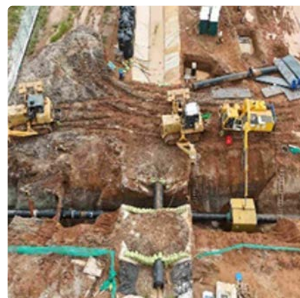
AGI-PPL Interface: 24" Pipe Welding Ongoing
