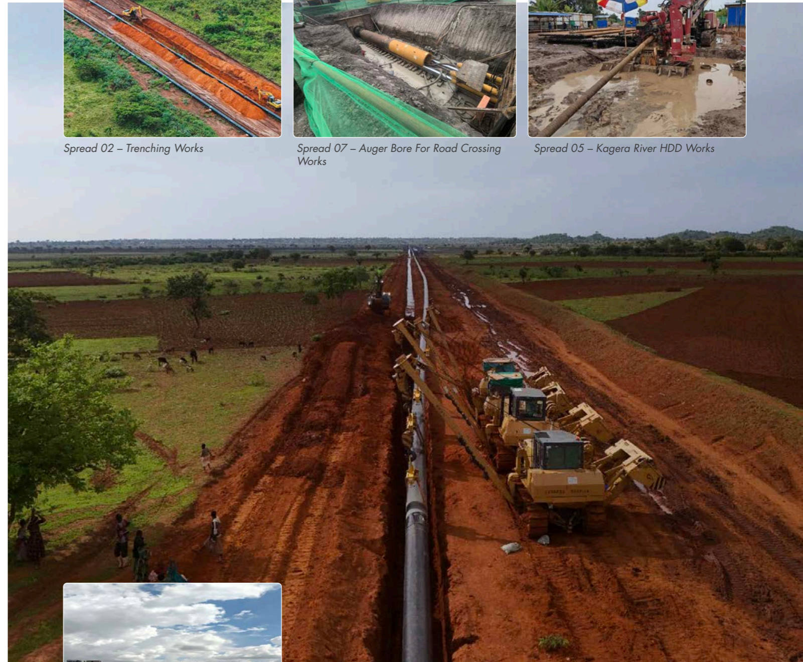
Spread 08 – Pipe Lowering Works
