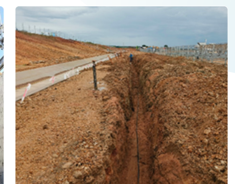
LV Cable Laying
