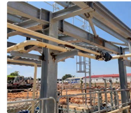
Pipe Support Erection
