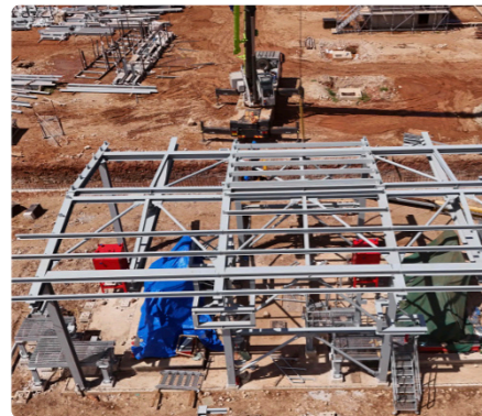
Fire Water Pump Shelter Installation
