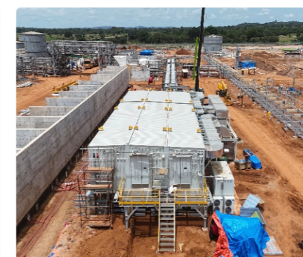
EITS Building HVAC Duct Installation
