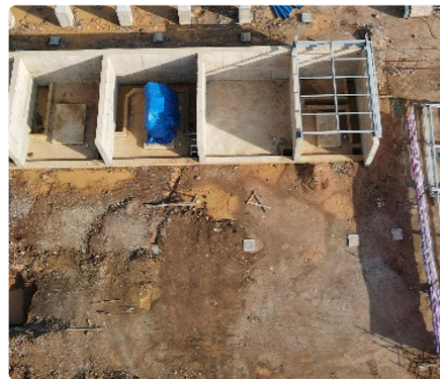
EITS Transformer Roof Installation
