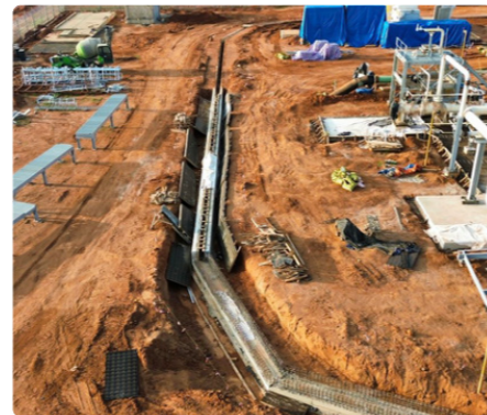
OD3 Concrete Trench Work
