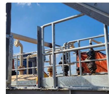
Steel Structure Platform Erection
