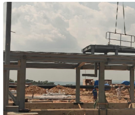
CDD Shelter Erection
