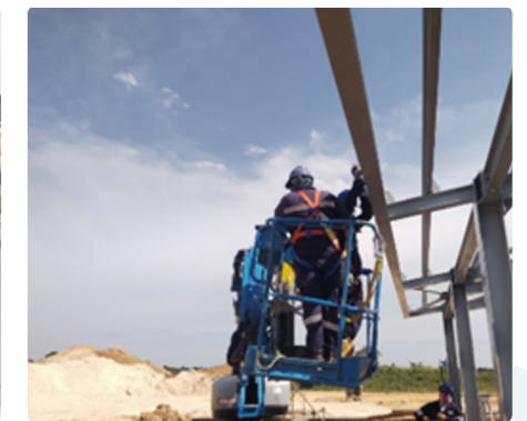
Steel Structure Bolt torquing
