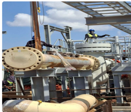
Export Pump B Suction Line Installation
