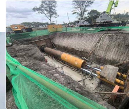
Spread 07 – Auger Bore For Road Crossing Works
