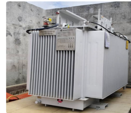
LLHT Transformer Installation
