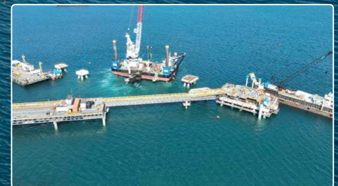
Dolphin Mooring Construction.
