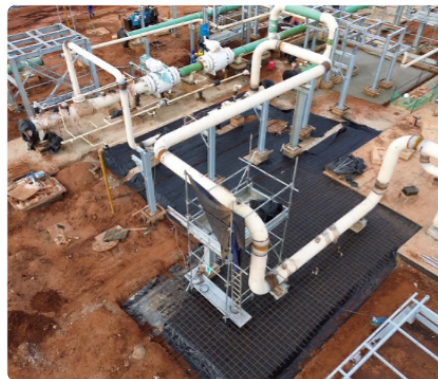
Rebar Paving Work
