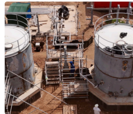
Cooling Water tank Piping Installation
