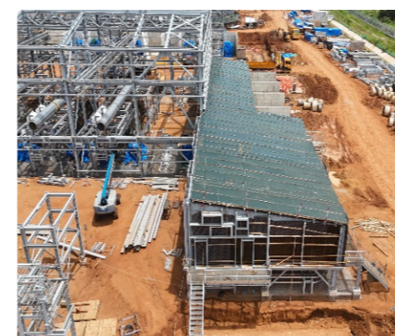
PGB: Elec Building Temporary Roofing ongoing
