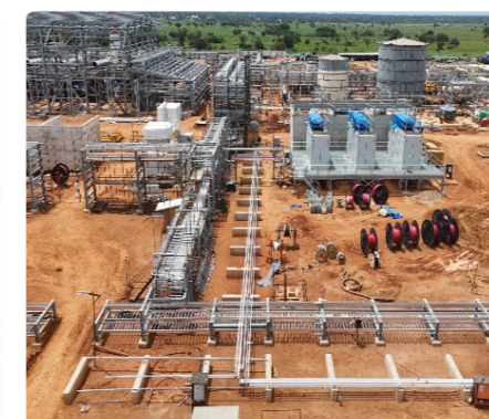
Utility Area Tray Installation and Piping Work
