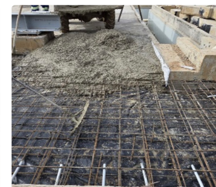
Process Area Paving
