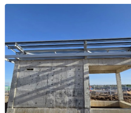
Guard House Roof Structure
