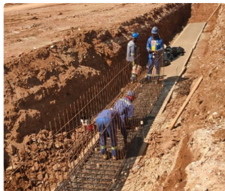
OD3 Trench Rebar Installation
