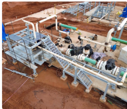
Pig Launcher Structure Installation
