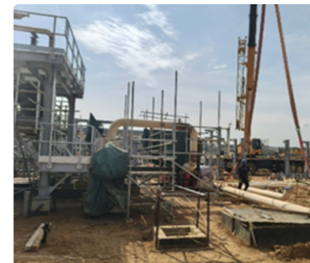
Piping Fit up
