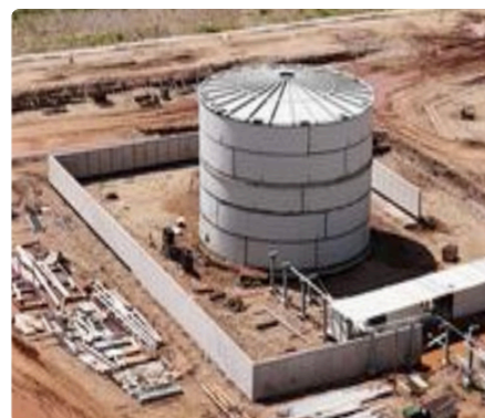
DFO Tank Bund Wall
