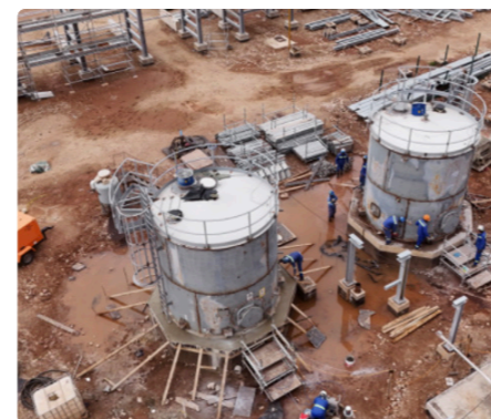
Cooling Water tank Inside Coating Completed
