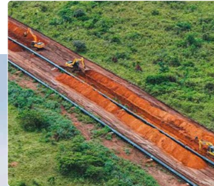
Spread 02 – Trenching Works
