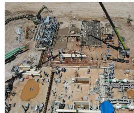
Process Area Paving
