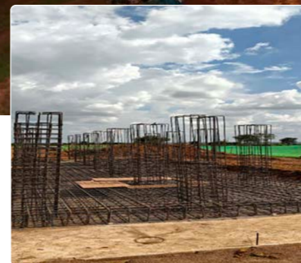
Spread 7 – MLBV-37 Reinforcement Installation works
