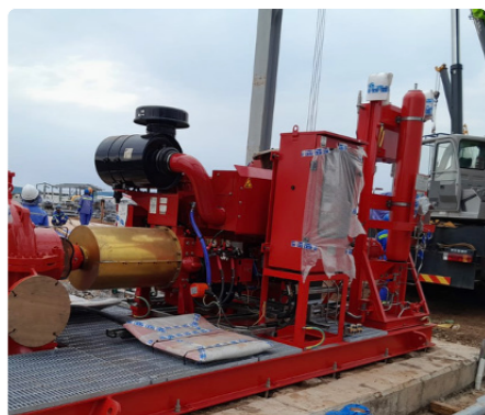
Fire Water Pump Installation
