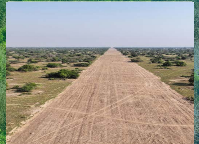
Restoration of the right of way.
