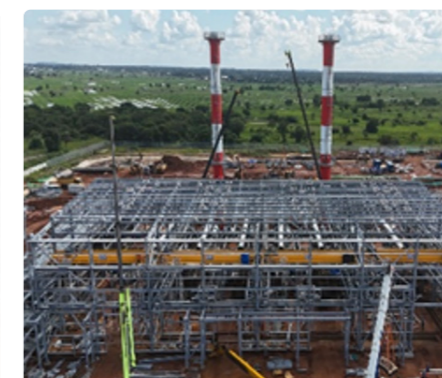
PGB-EOT Crane Installation
