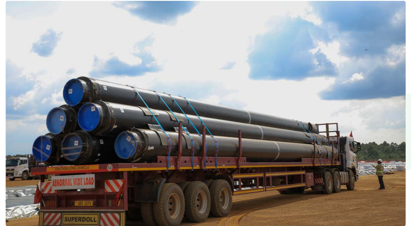
EACOP Pipe transportation.
