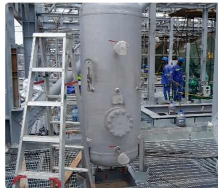
PGB Air Receiver Installation
