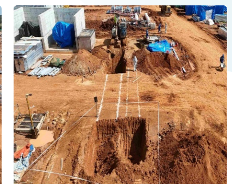
EITS Area Cable Trench Excavation
