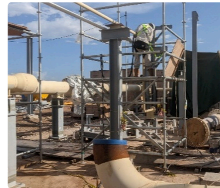
Process Area Piping Erection
