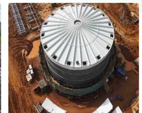
FW Tank: Shell Plate erection & welding ongoing
