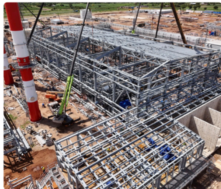
PGB Steel Structure Erection
