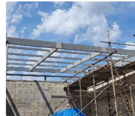
Steel Structure Installation
