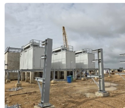
VSD E House Structure Installation
