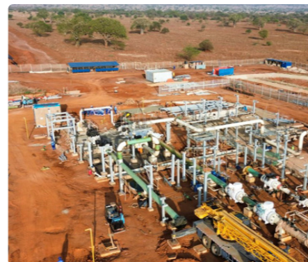
CPS & CTS Installation
