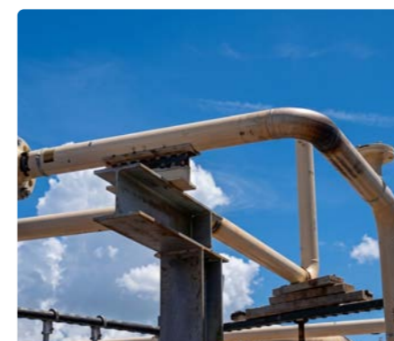
Pipe Support Erection
