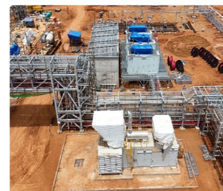
Cable Tray installation
