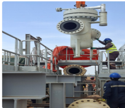
Export Pump A Suction Line Installation
