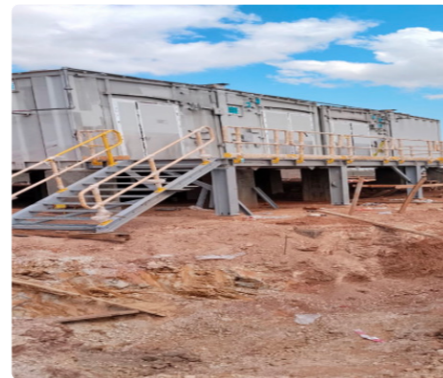
66kV Platform Handrail Installation
