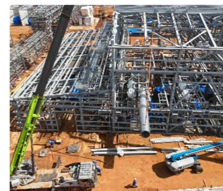
PGB: Installation of Exhaust Ducts for GENSET-A
