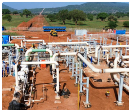
Piping Spool Installation
