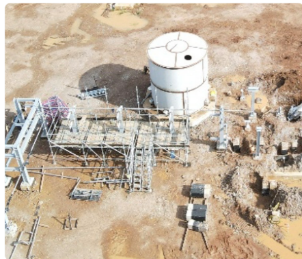
Steel Structure Platform Installation
