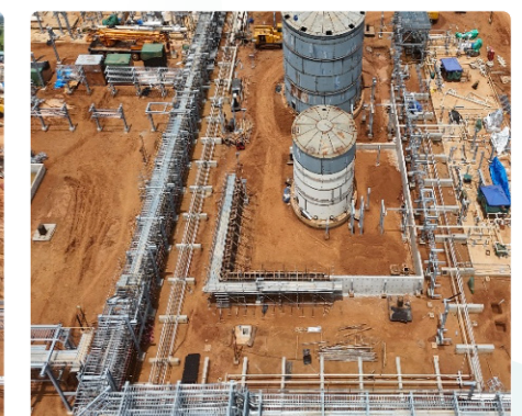
CFO Tank Bund Wall and Piping Installation
