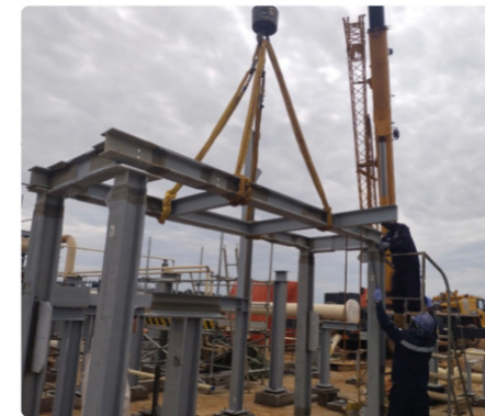
Steel Structure Installation
