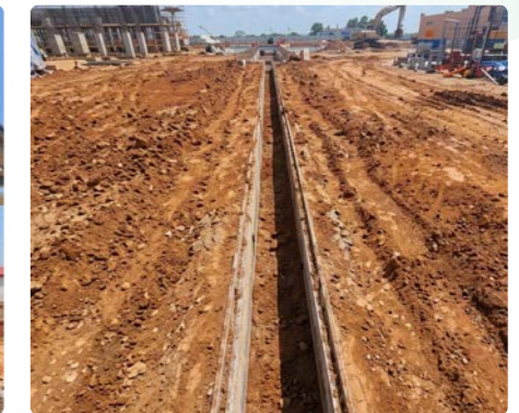
OD3 Trench Backfilling
