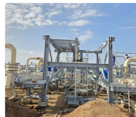
Receiver/ Launcher Structure Erection
