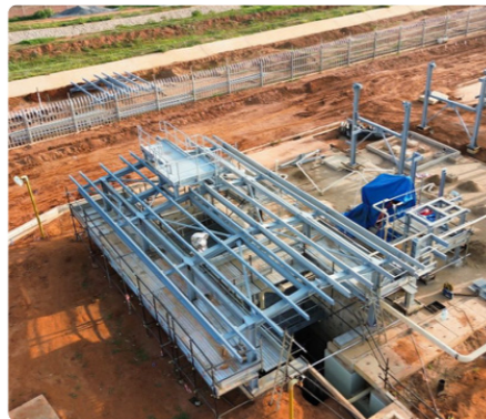
CDD Structure Installation
