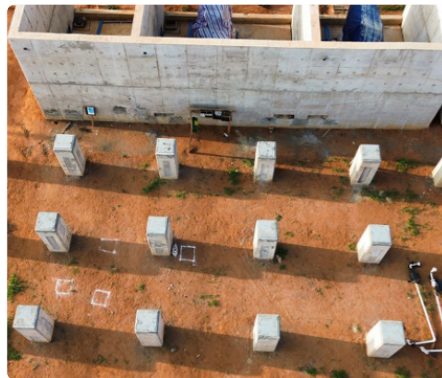
EITS Foundation Plate Works
