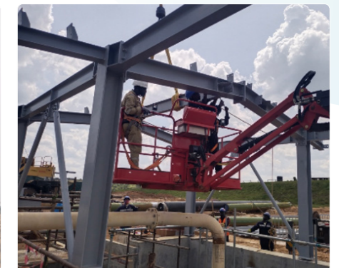
CDD Shelter Structure Installation
