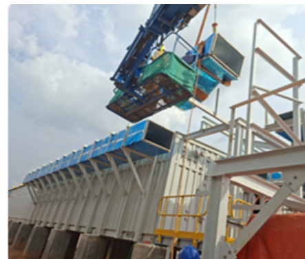
66kV Platform Handrail Installation
