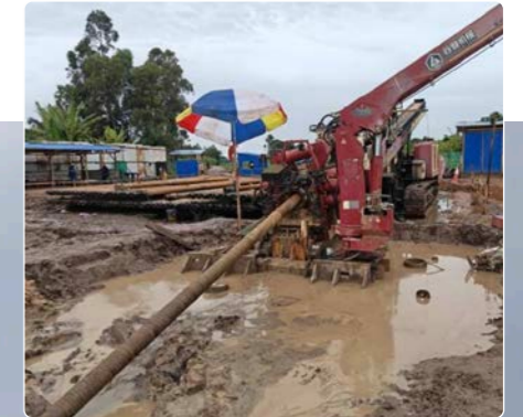
Spread 05 – Kagera River HDD Works
