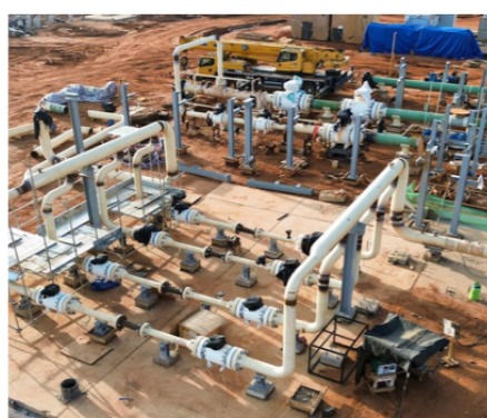
Process Area Piping Installation
