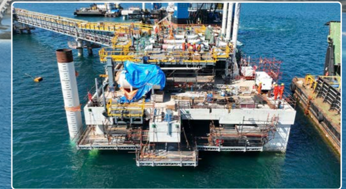
Load out Facility (LOF) works and form-scaff installation.
