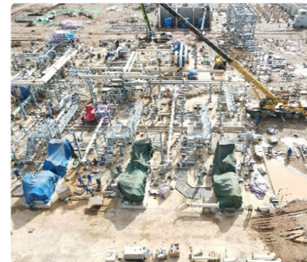
Process Area Piping Installation
