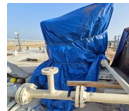
Re Injection Pump Pipe Welding
