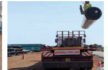
Loading coated pipes ready to dispatch to MCPYs in both countries - TZ & UG.
