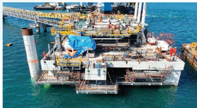
LOF works and form-scaff installation.
