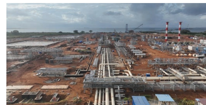
Along C1 pipe sleeper (from JETTY to tank).
