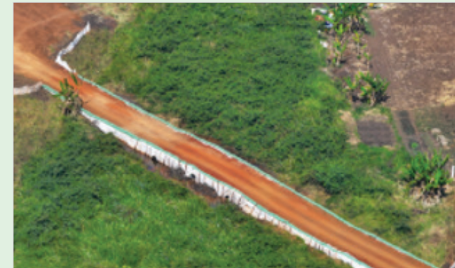
Cearing and grading of the Right of Way (RoW).
