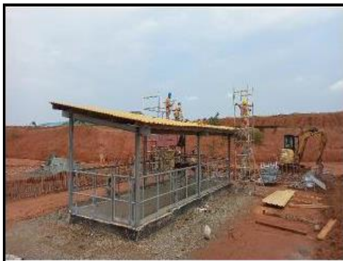
Figure 15: JBR03 - Installation of Roofing Sheets on Emergency Pit
