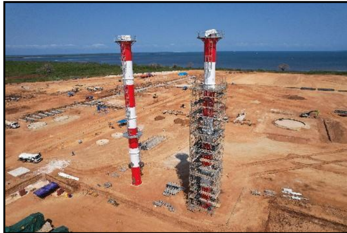
Figure 8: Marine Terminal Exhaust Stack (Source: EACOP Monthly report. October 2024).
