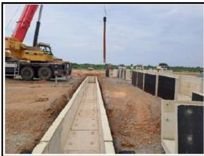
Figure 14: KAS01 Well pad - Technical Culvert Installation at Tubular Handling Area
