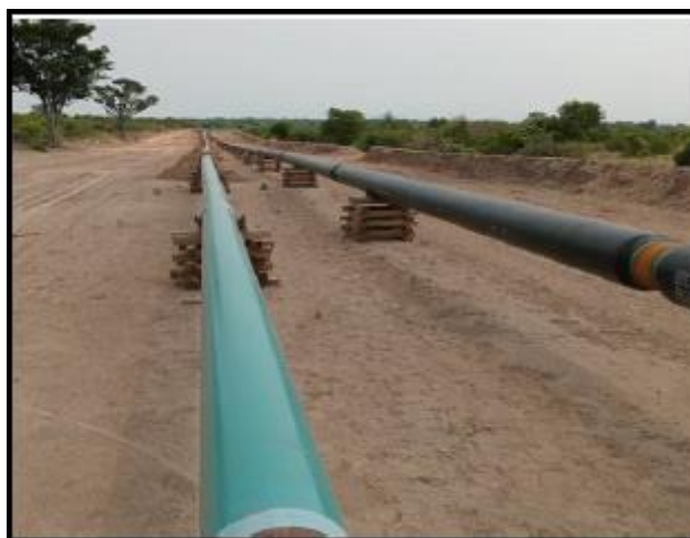
Figure 19: NGR05 - CPF Oil Flowline welding and stringing
