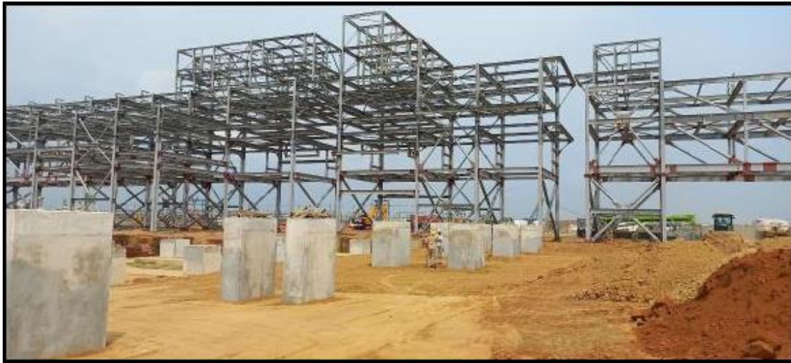
Figure 17: CPF: Oil Treatment 1 foundation back-filling
