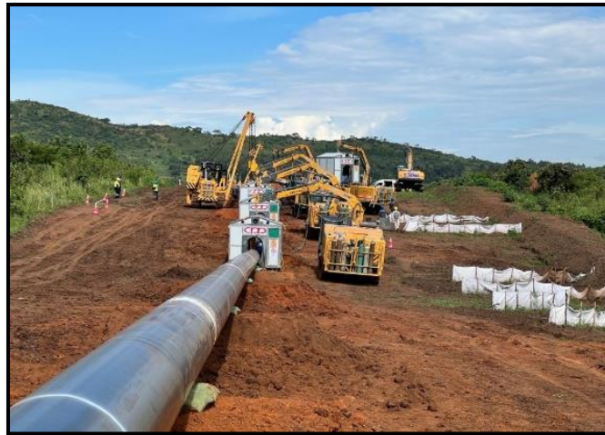
Figure 6: Lot 1 – pipeline welding (Source: EACOP Monthly report. October 2024).
