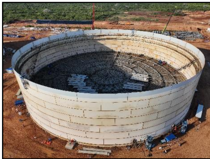
Figure 9: Marine Tank B – 7 th shell plate erection (Source: EACOP Monthly report. October 2024).
