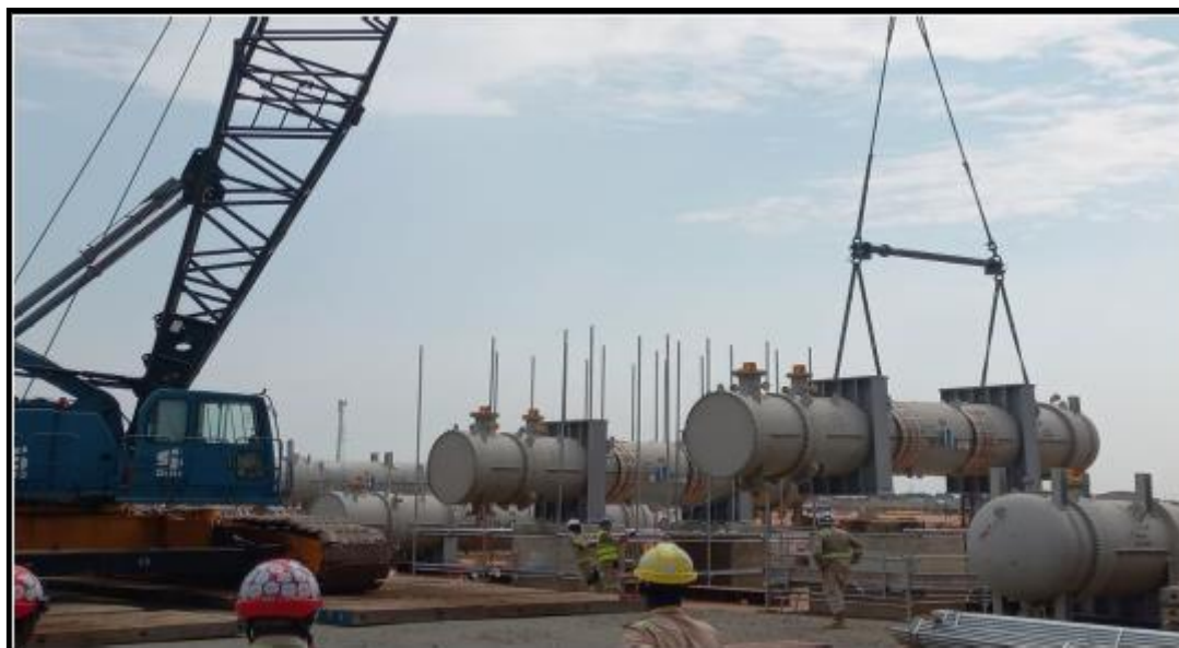
Figure 21: CPF: Pre-heaters lifted and positioned on foundations
