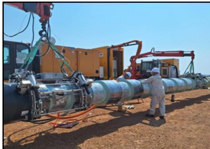
Figure 7: Lot 3 – field joint coating pre-production test (Source: EACOP Monthly report. October 2024).
