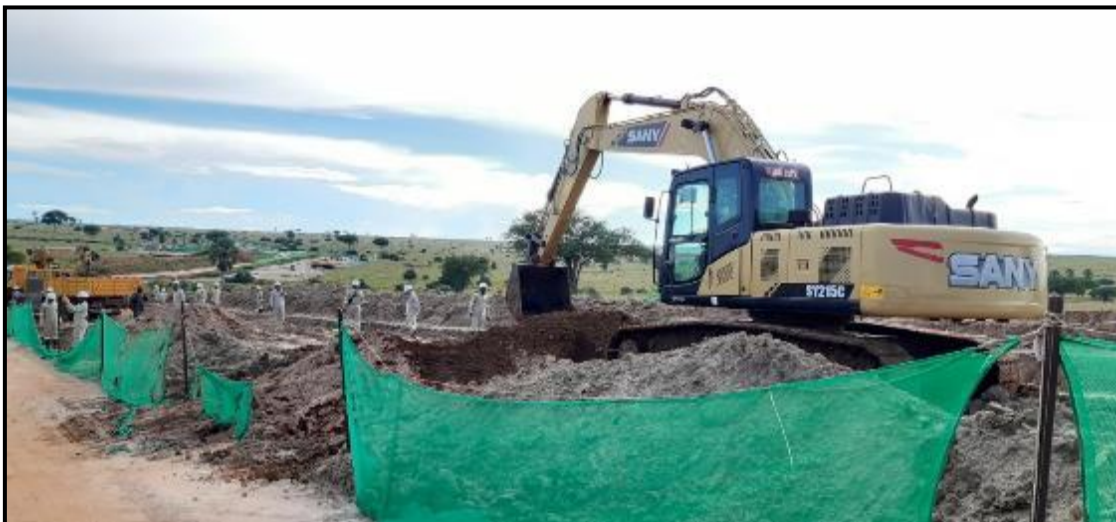
Figure 15: Flow Lines for Tilenga under construction (Source: LESC Field Visit, November 2023).
