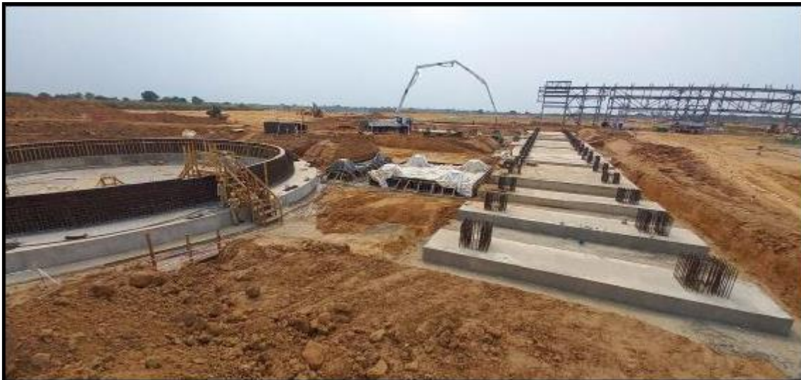
Figure 18: CPF: Water Injection Tank and Pipe Rack Foundations
