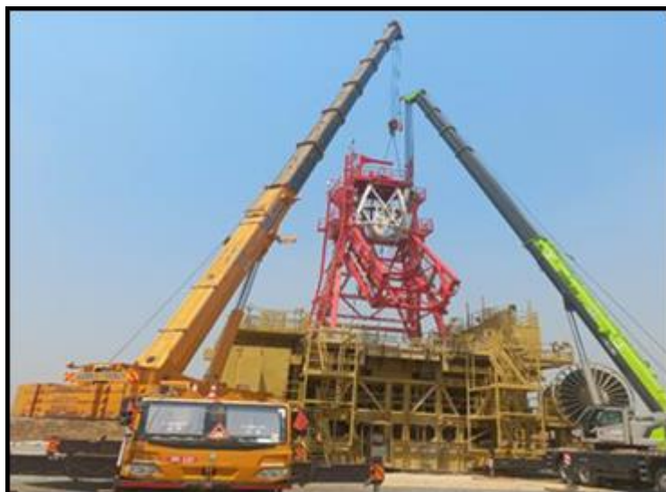
Figure 16: JBR05: Rig-down of mast
