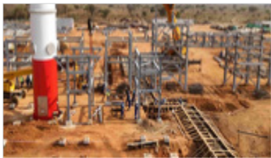
Exhaust Ducts & Cable Tray Supports Erection Started.
