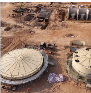
CFO Storage Tank roof welding ongoing.
