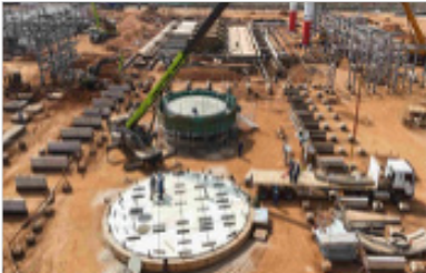
CFO Storage Tank: Base Plate Erection Ongoing.
