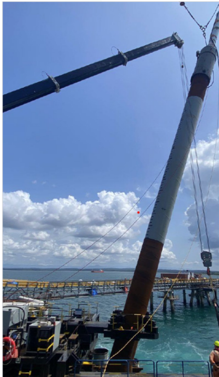
5. Impact driving (using S-150 hydraulic hammer).
