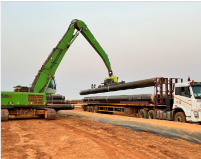
TIS yard - Ongoing PUF pipes load-out on MLC trucks to be shipped to MCPYs.
