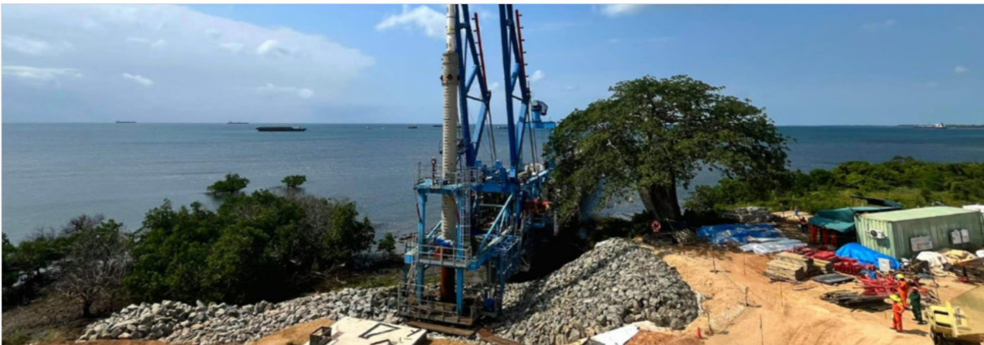
The launching girder has reached the abutment and installed the last 60 piles.
