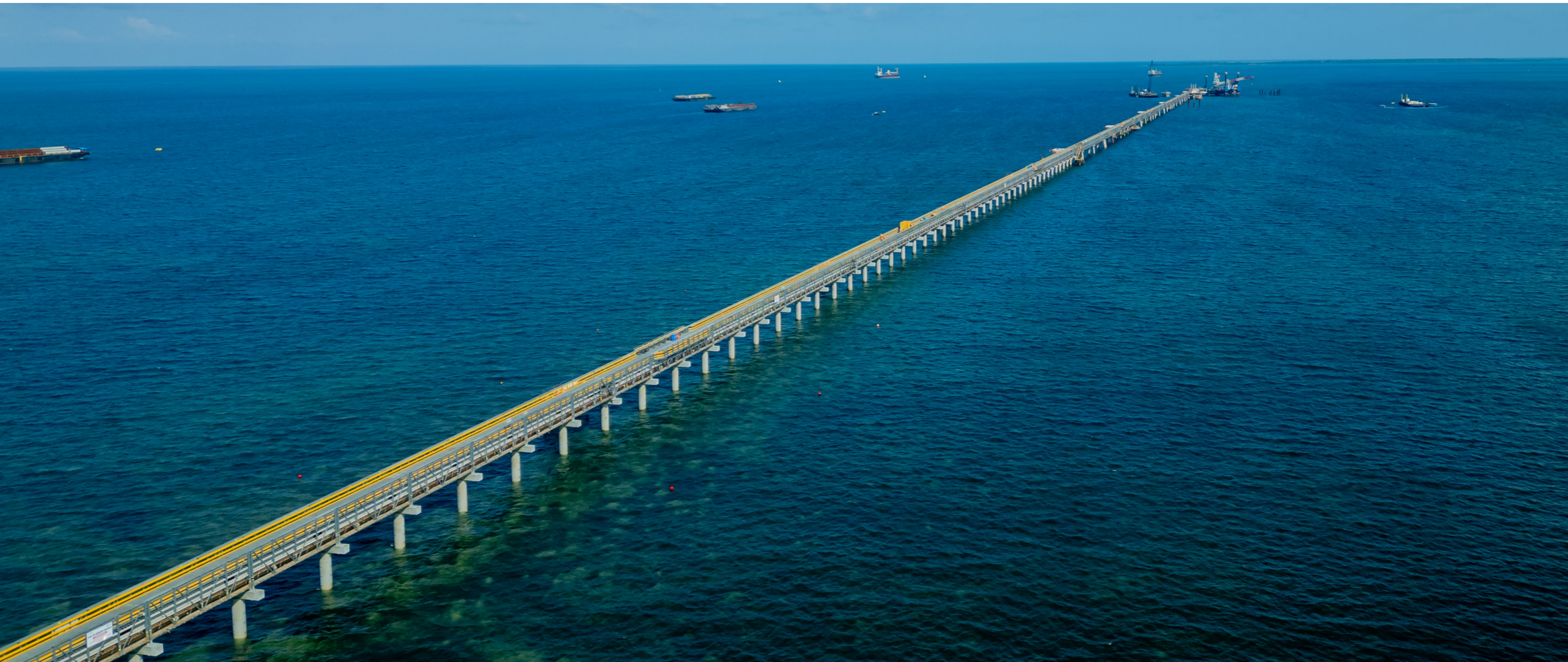
Installation of the last truss by RIMA jack-up barge. The nearly 2 KM long trestle is now completed and the LOF platform is connected to the shore.
