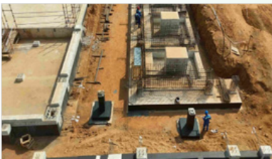
PG Transformer Bay: Rebar installation for Walls ongoing.
