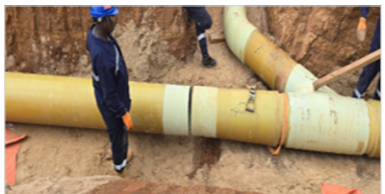
GRE Pipe installation.
