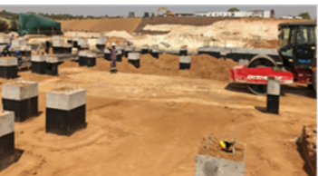
CTS & CPS near CDD Back filling, compaction in progress.
