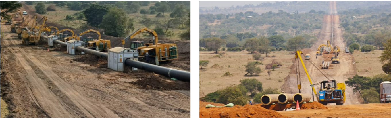
Pipeline installation works are underway in Spread 3-LOT 1, Uganda, featuring side booms aligning and lowering of pipeline sections into the trench. Photos illustrate right-of-way preparation, pipe stringing, welding, coating, and lowering operations as part of the ongoing EACOP project.
