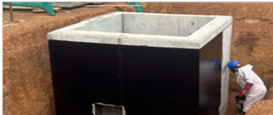
Bitumen coating for valve pits ongoing.
