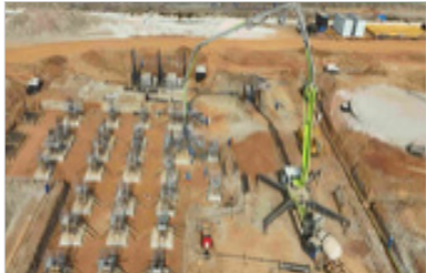
Office Building FND: Concrete Casting Ongoing.
