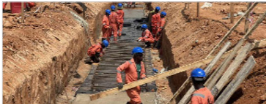
Steel fixing for Concrete fence in progress.
