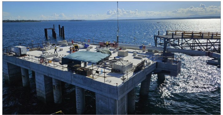
Concrete casting for second layer and pedestal completed
