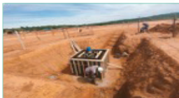
Manhole Formwork Installation
