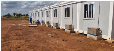
MCPY7 - installation of outdoor AC units
