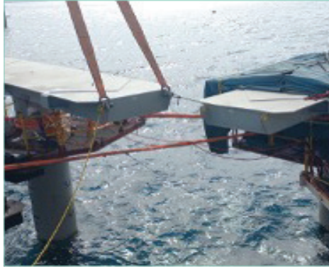
Crosshead Installation for loop
