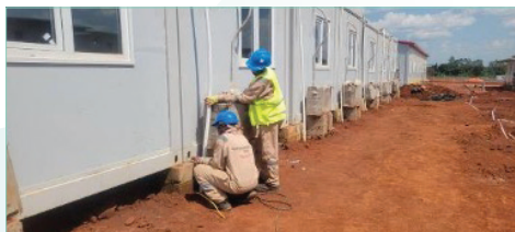
MCPY1 - fixing earthing cables
