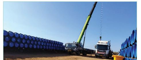
MCPY11 - pipe delivery to the row
