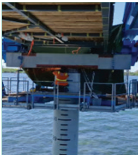
2. Cross Head Installation/welding
