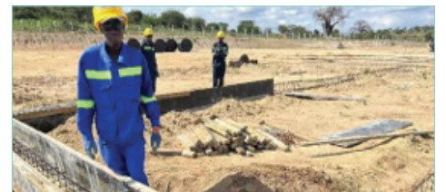
MC12 & PY12 concrete foundation FPR CTR canteen type 1
