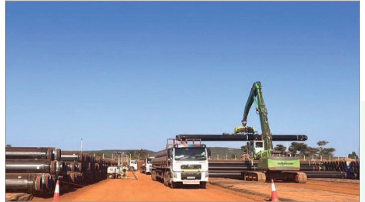
Loading coated pipes ready to dispatch to MCPYs
