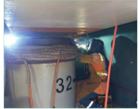
Welding X-head to pile
