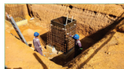
Formwork Installation for Sanitary Manhole 1007
