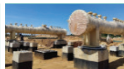
Pig Launcher & Receiver Installation
