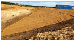
Erosion Mating Installation
